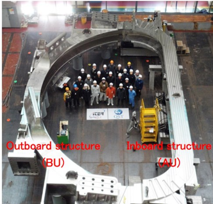
Fitting test of the 1st TF Coil Inboard and Outboard structures at Hyundai Heavy Industries
